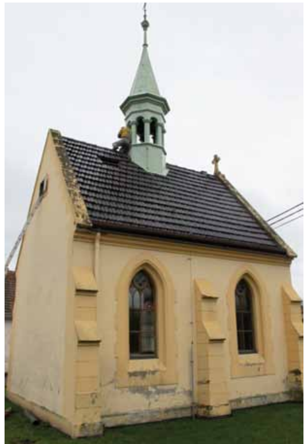
The chapel with a serviceman on the roof inspecting the bell.
