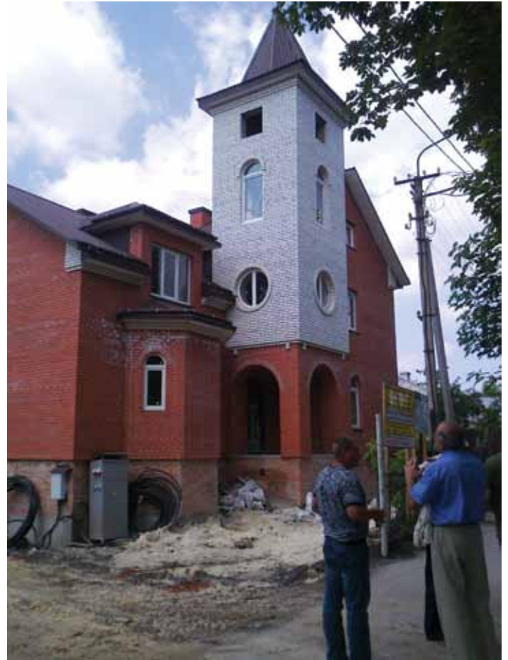
Church under construction in Ternopil.
